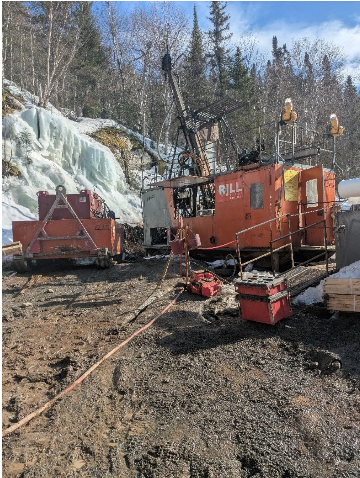
Figure 12.6: Active Drill Rig at Geminid
